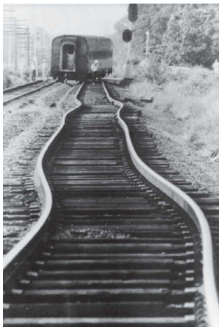
FIGURE 21-6. Railroad tracks distorted because of thermal expansion on a very hot day. Railroad tracks today come in 1500-ft lengths and, to prevent buckling, are laid at or near the maximum annual temperature of the locality.
